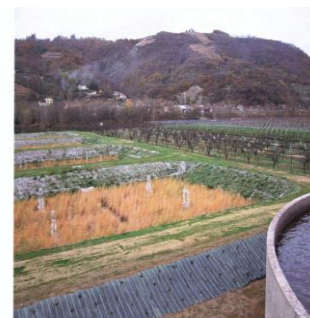
Reed beds for sludge treatment
